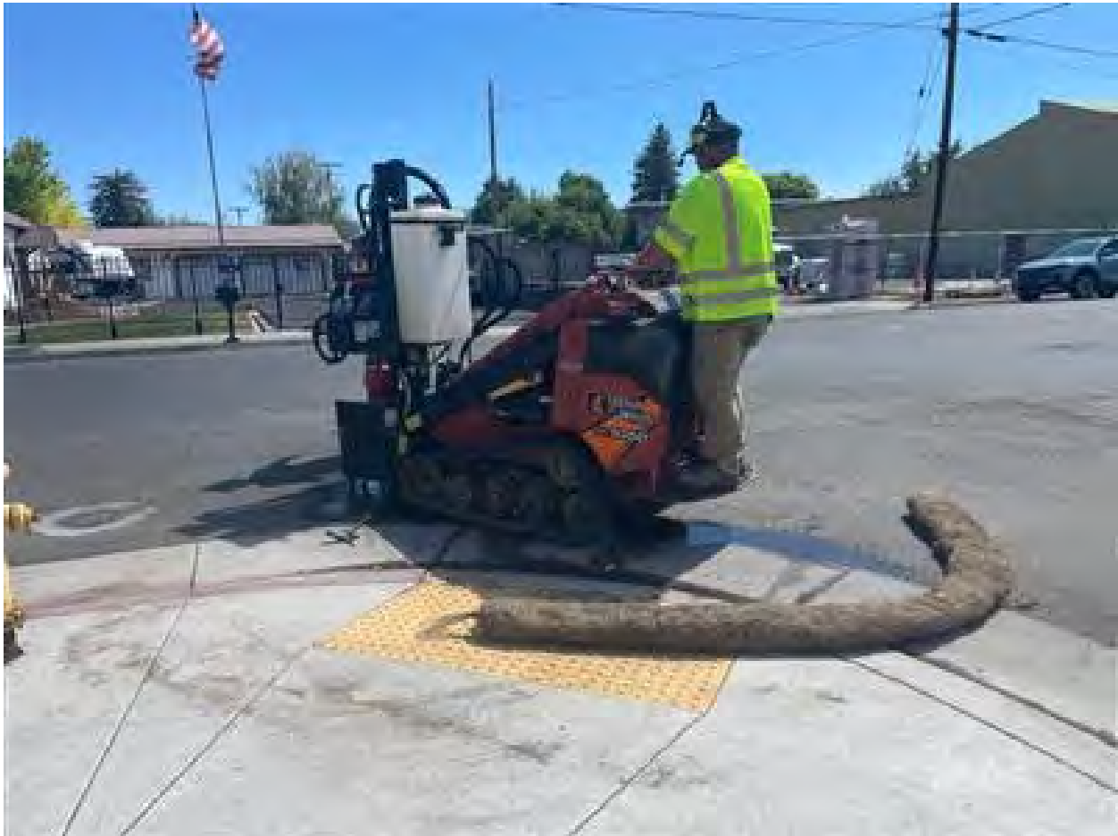
Figure 14. HDD equipment with straw waddle (BMP).
