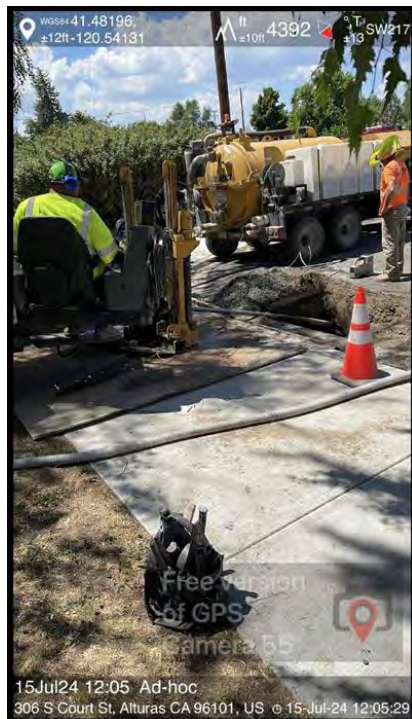
Figure 6. View to the southwest of HDD work in Alturas.
