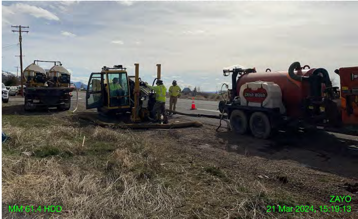
Figure 15. HDD equipment with straw waddle (BMP) and Vac-Truck.
