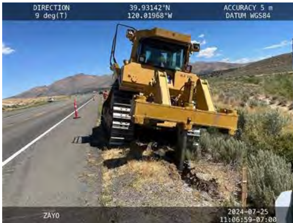
Figure 10. View to the north of pre-ripping crew in the Southern Area (Lassen County).
