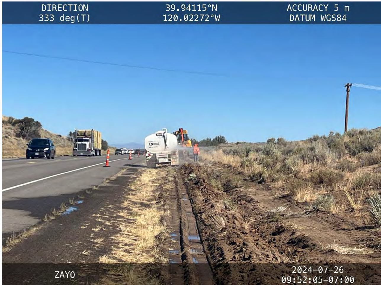
Figure 13. Laying conduit while using the water truck for dust
