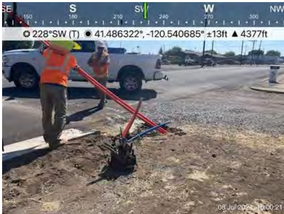
Figure 2. View to the southwest of Central Area drilling crew in Alturas.
